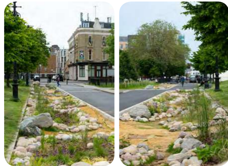
Exemplar Bioretention System specific to public realm example. Shoreditch, London
