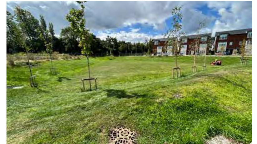
Figure 25: Detention Basin – Kilgobbin, Dublin
