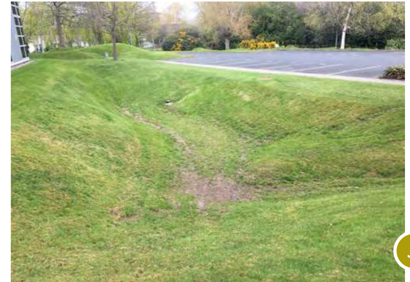
Figure 14: Detention Basin - City West, Dublin
