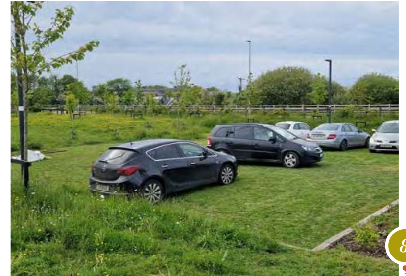
Figure 20: Proprietary Reinforced Grass - Min Ryan Park, Wexford
