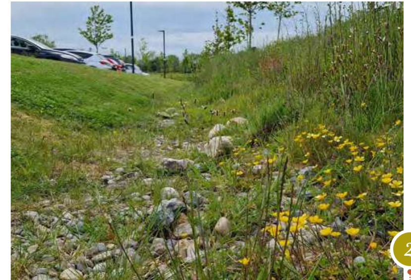
Figure 8: Dry Swale - Min Ryan Park, Wexford
