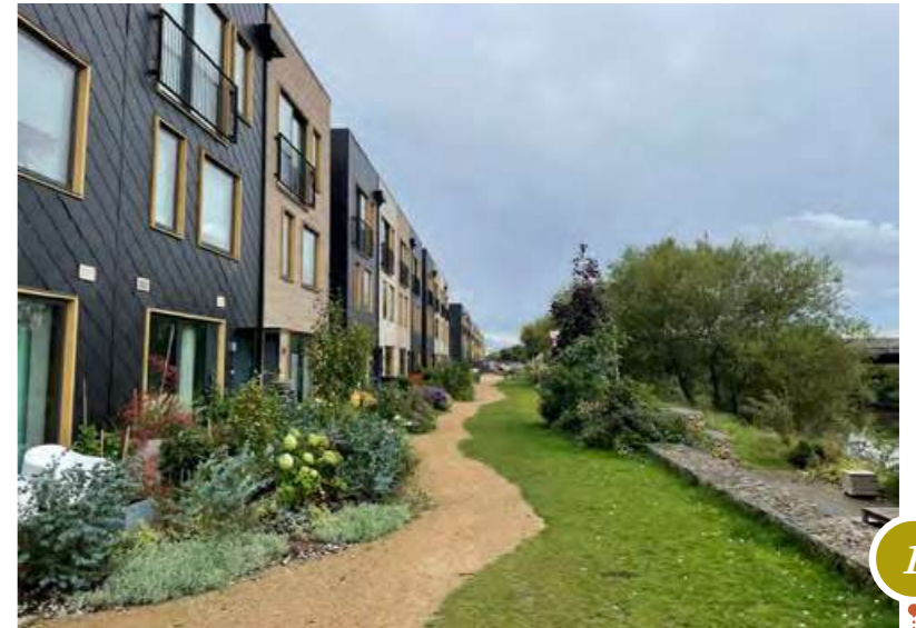
Figure 6: Filter Drain - Climate Innovation District, Leeds
