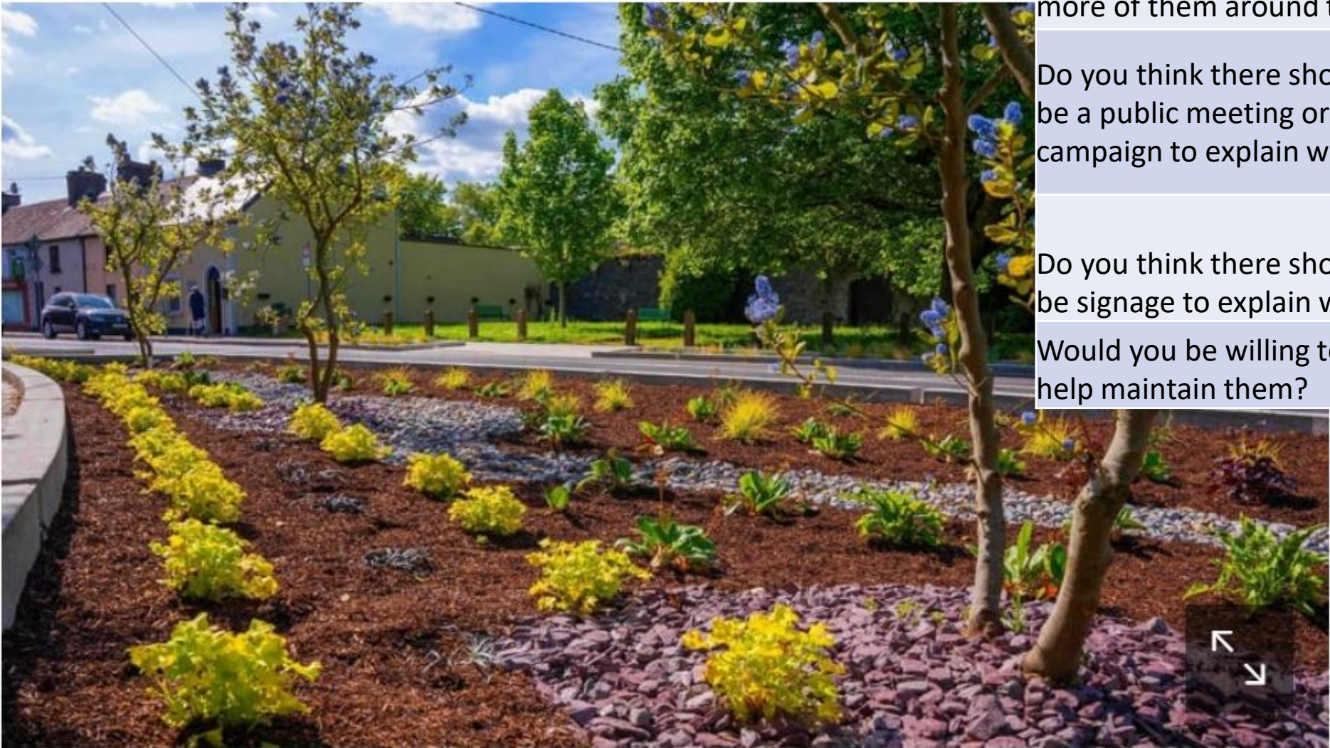
Carlow's rain gardens are a free draining soil mix that cleans, stores and conveys runoff water
