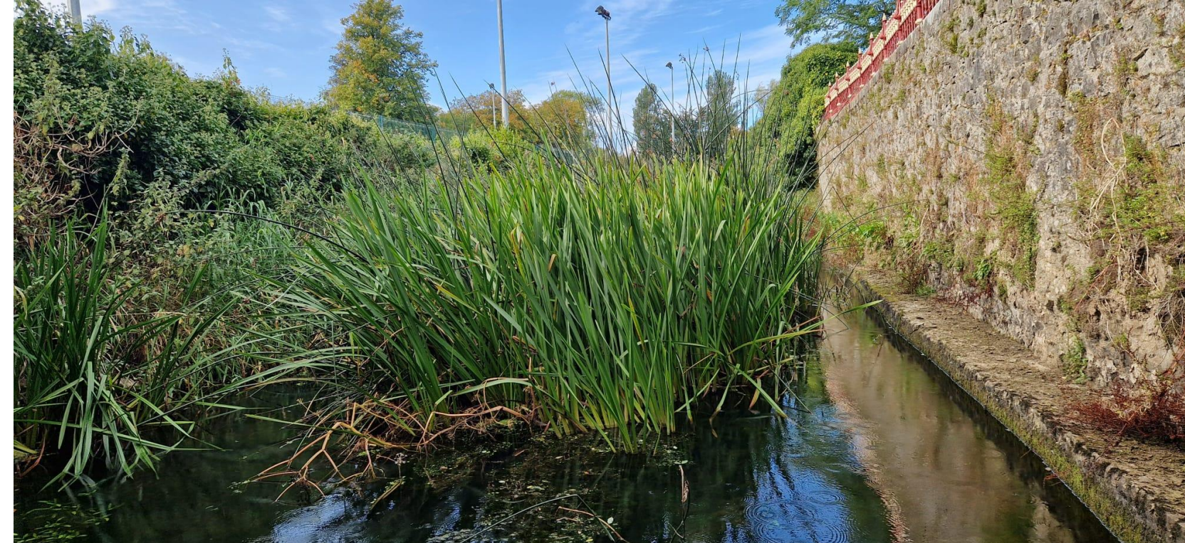
High level of silt (below) and river plant growth evident (above) upstream
