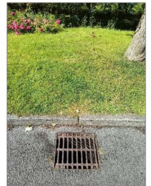
Storm grate diverting road runoff into Athlone Canal
