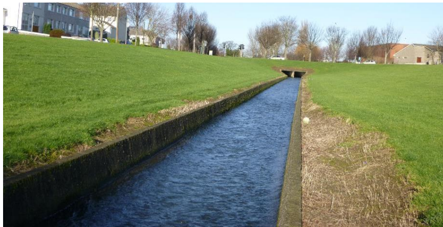
Figure 20: Example of culverted section of river
