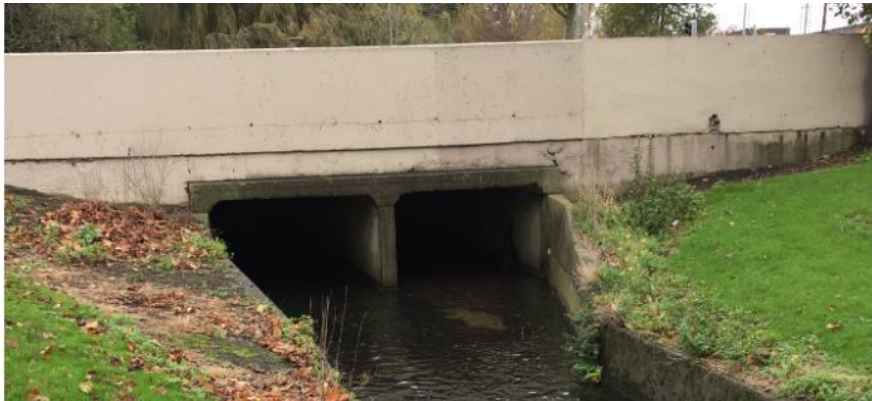
Figure 23: Example of Culverted Bridge
