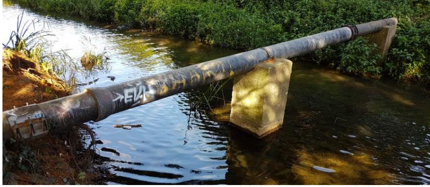
Figure 21: Example of Pipe Support across River
