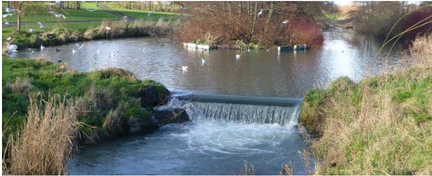
Figure 22: Example of "Ornamental" Weir
