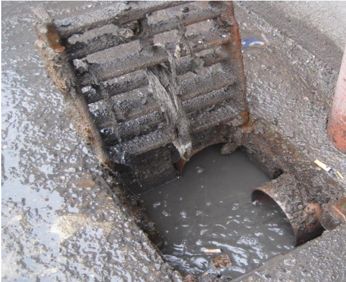
Figure 11-6: Surface water gully receiving polluting matter as contaminated runoff from industrial premises yard. (Photo: Emmet Conboy).
