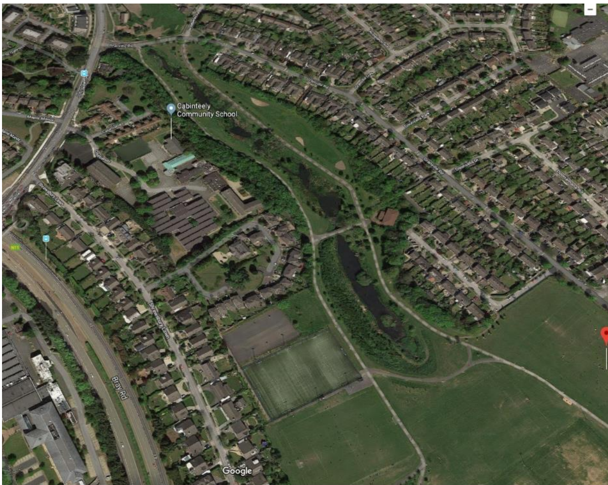
Figure 5-10: Kilbogget Park Integrated Constructed Wetland on the Deansgrange River treating surface water impacted by urban pressures – primarily misconnections. MRP (mg/l) is halved from inlet to outlet of the wetland. (Photo: Google Maps).
