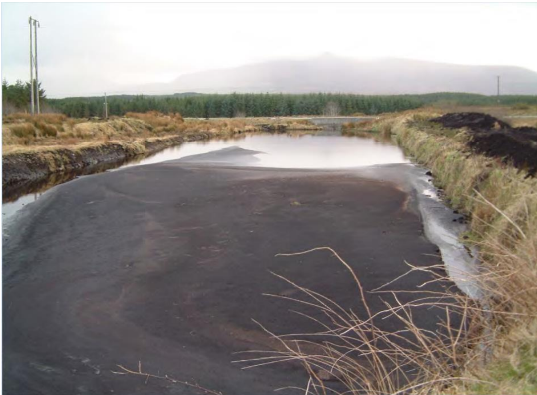
Figure 8-7: Silt (settlement) pond at Bellacorrack Bog, Co. Mayo (Copied from Kennedy et al., 2012).
