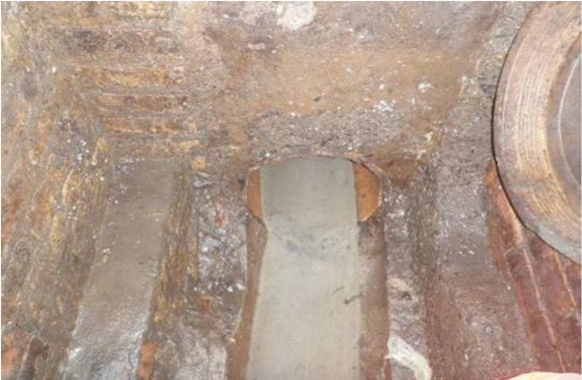
Figure 4-12: Typical SWO. Normal flows run in the channel. When levels rise in the manhole, excess flow escapes via the overflow pipe to the right of the photo (Photo: Paul Buggy & Gerry O'Connell).
