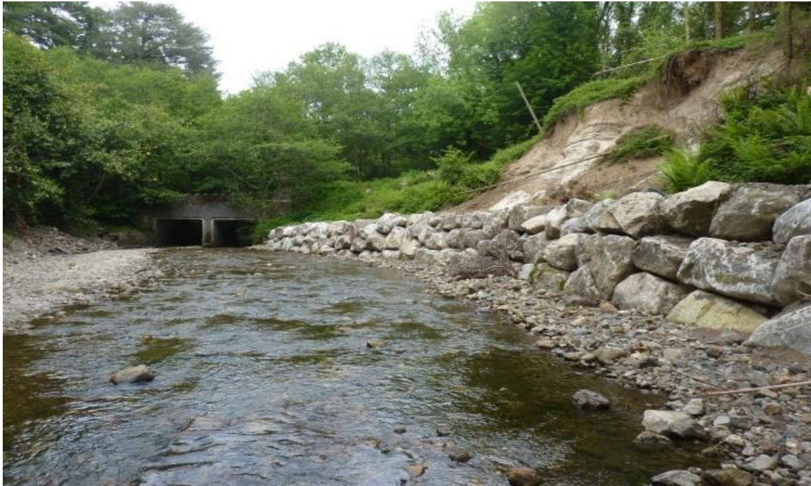
Figure 3-9: Example of the use of boulders as bank protection. By placing boulders along the river bank, this prevents lateral movement and in response, the river may erode the banks elsewhere (Photo: Emma Quinlan).
