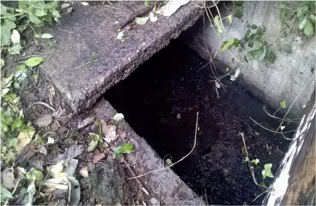
Figure 6-7: Bad Practice – Open tanks which allow ingress of rainwater into the system and constitutes a risk to human health (Photo: Joan Martin).
