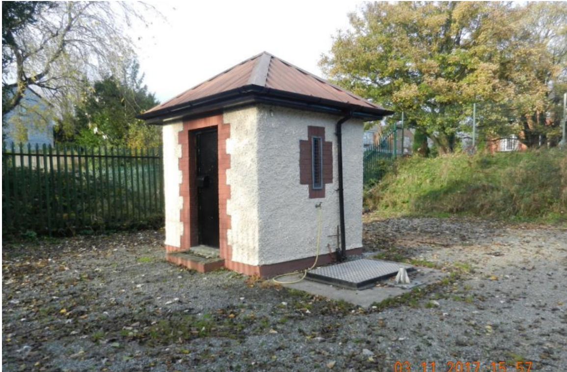
Figure 4-18: Typical foul pumping station compound & control building (Photo: Joan Martin).
