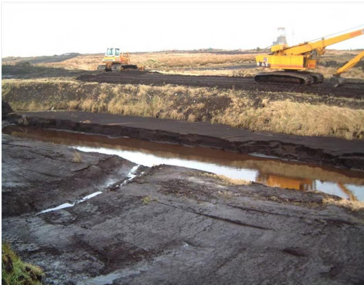
Figure 8-8: A silt pond west at Bellacorick Bog in the process of being emptied in 2002 (Photo copied from Kennedy et al., 2012).
