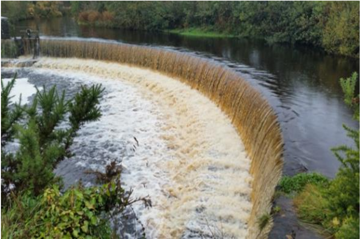
Figure 3-4: Example of a weir. This structure will impact the movement of bed load material (e.g. sand, gravel, cobble and boulders) and impact flow conditions directly upstream and downstream of the structure. It will also impede the movement of aquatic species. A fish pass is present on this weir (not visible in the photo) but it is not functioning (Photo: Emma Quinlan).
