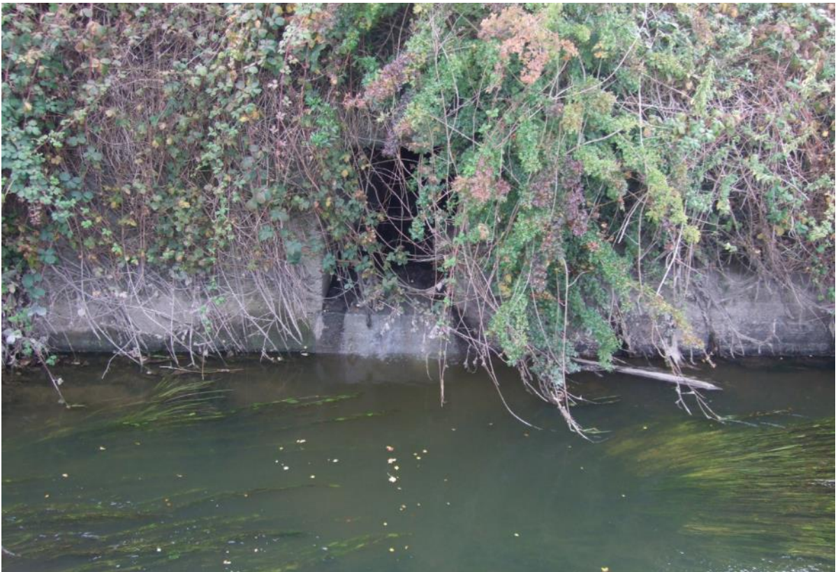
Figure 4-13: Example of a SWO on a combined network in dry weather – Note the evident eutrophication (Photo: Joan Martin).
