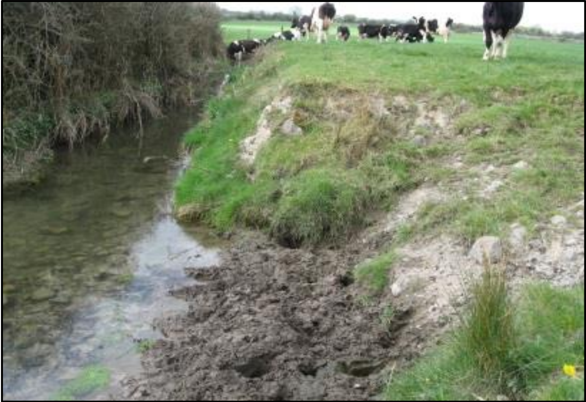
Figure 2-26: Bank erosion caused by cattle access (Photo: Robert Imbusch).
