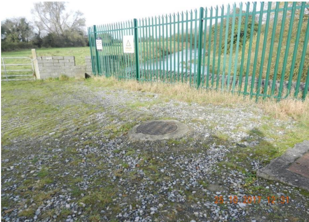
Figure 4-4: Note, manholes downgradient of treatment plant can indicate the discharge locations which may be under the surface water level of the receiving water (Photo: Joan Martin).
