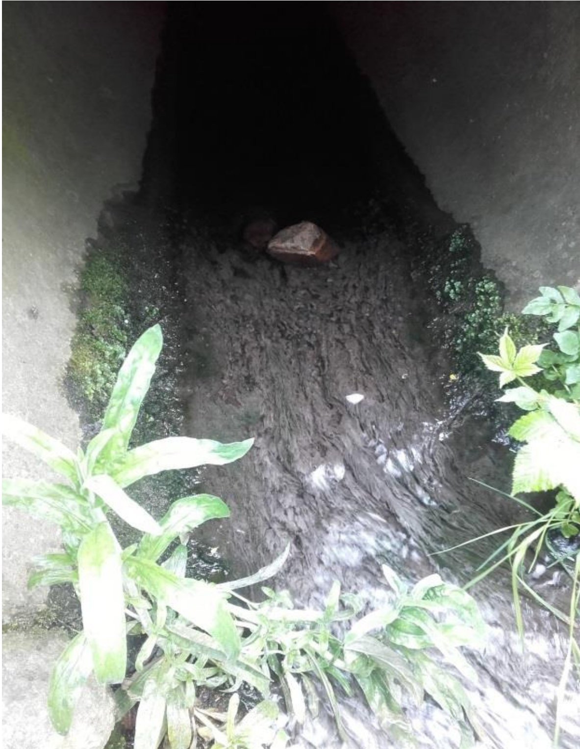
Figure 5-9: Sewage Fungus within a surface water pipe showing evidence of misconnections (Photo: Paul Buggy).
