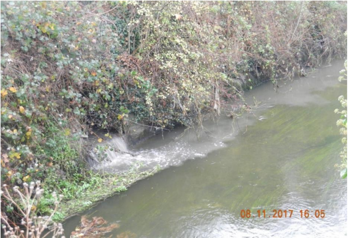
Figure 4-14: Bad Practice – Example of a SWO on a combined network in wet weather. Note the contaminated overflow into the receiving water in moderate rain conditions (Photo: Joan Martin).
