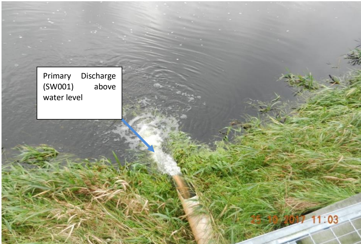
Figure 4-7: Primary Discharge. Note the continuous flow and discharges should be clear with no visible solids (Photo: Joan Martin).
