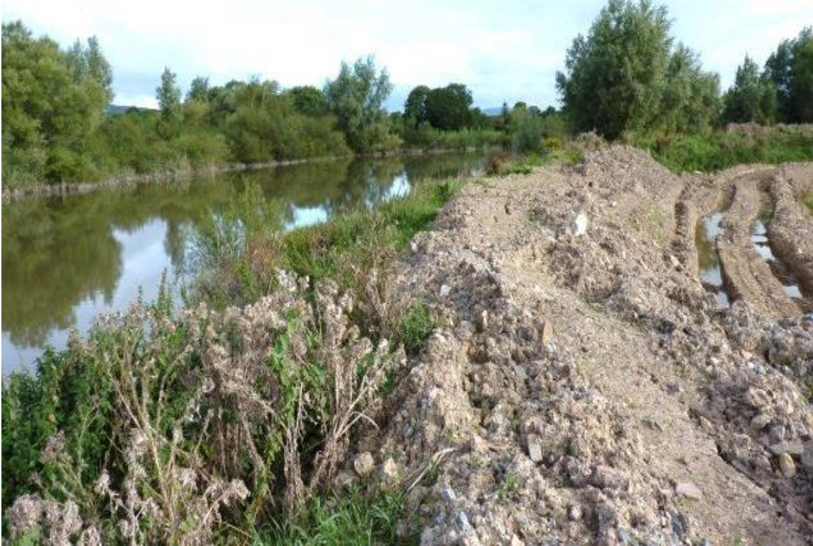
Figure 3-12: Example of the use of embankments as flood protection. Note the spoil heaped onto the bank has disconnected the channel from its floodplain. If soil is bare, this can act as a sediment source (Photo: Emma Quinlan).
