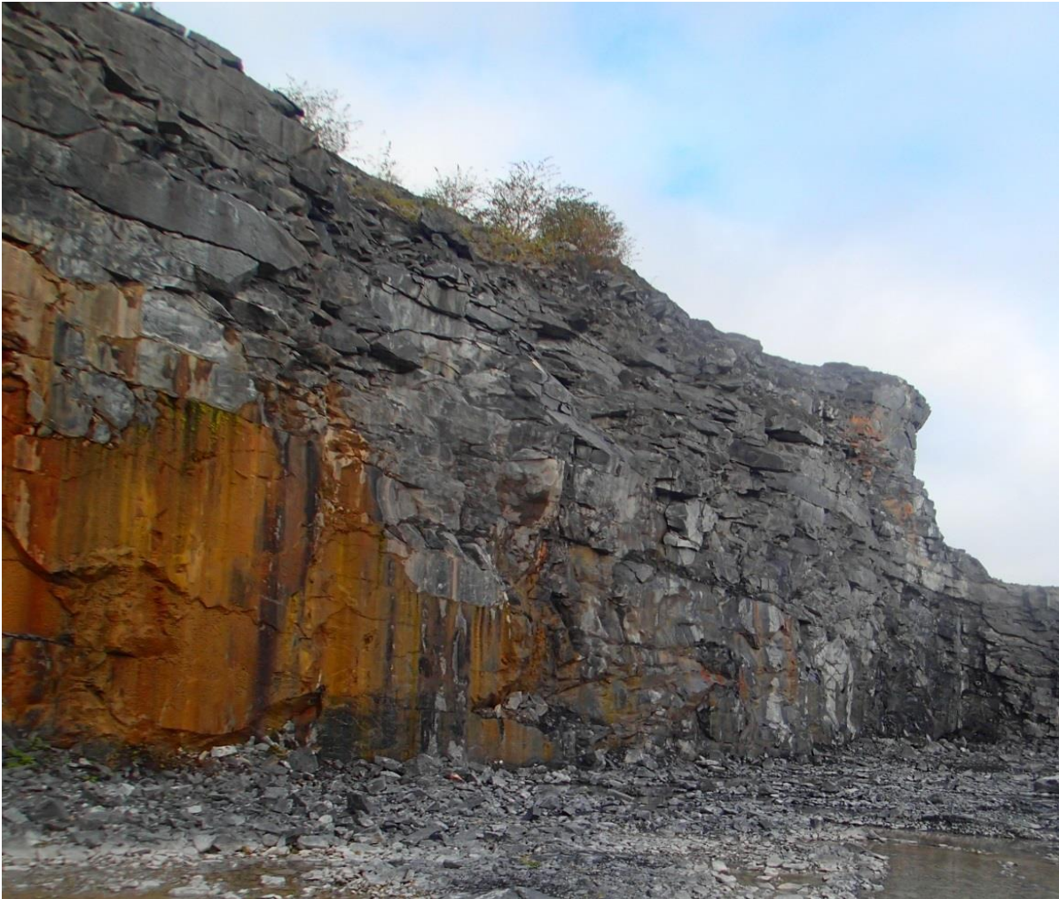
Figure 5-6: Seeps at bedding planes in quarry (shown by orange streaks) (Photo: Robbie Meehan).
