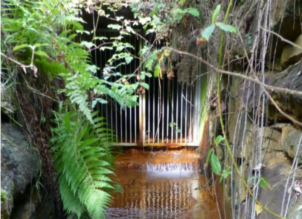
Figure 10-1: Acid mine drainage from the Deep Adit at the Avoca Mine, Co. Wicklow (Photo: Pat Barrett).
