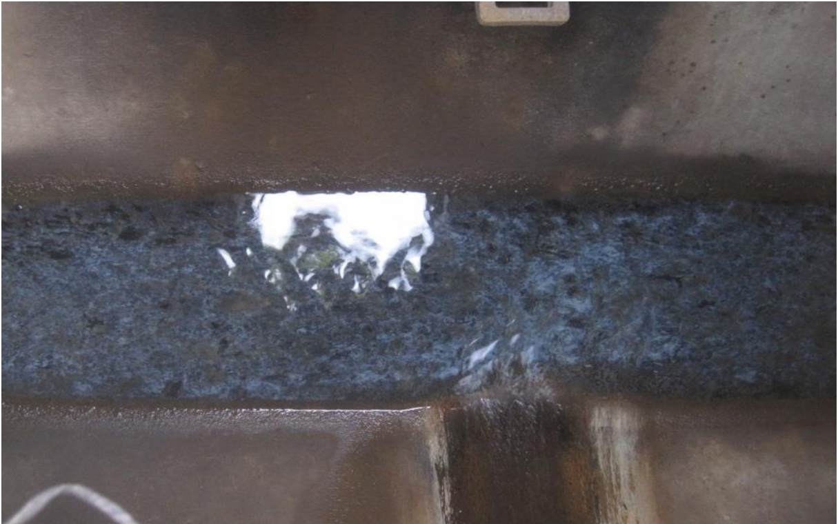
Figure 11-2: Storm drain with indication of polluting inputs – sewage fungus at base of drain (Photo: Emmet Conboy).
