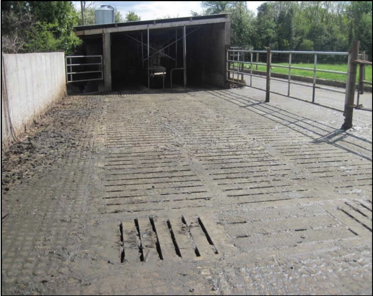
Figure 2-4: Slatted tank (Photo: Andrew Holmes).
