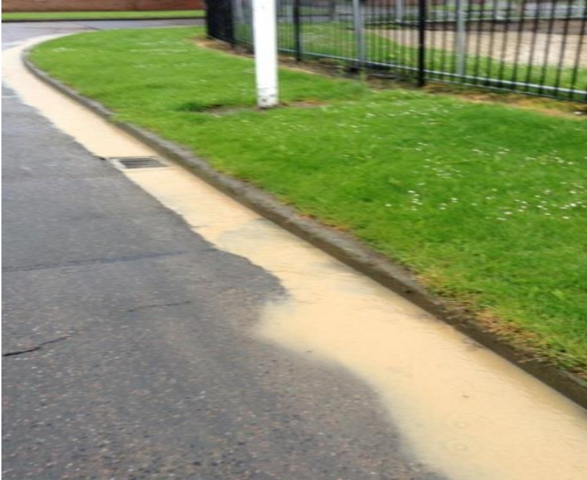
Figure 5-15: Pumped water from a road trench making its way to the surface water gullies and then to the local stream (Photo: Gerry Cullen).
