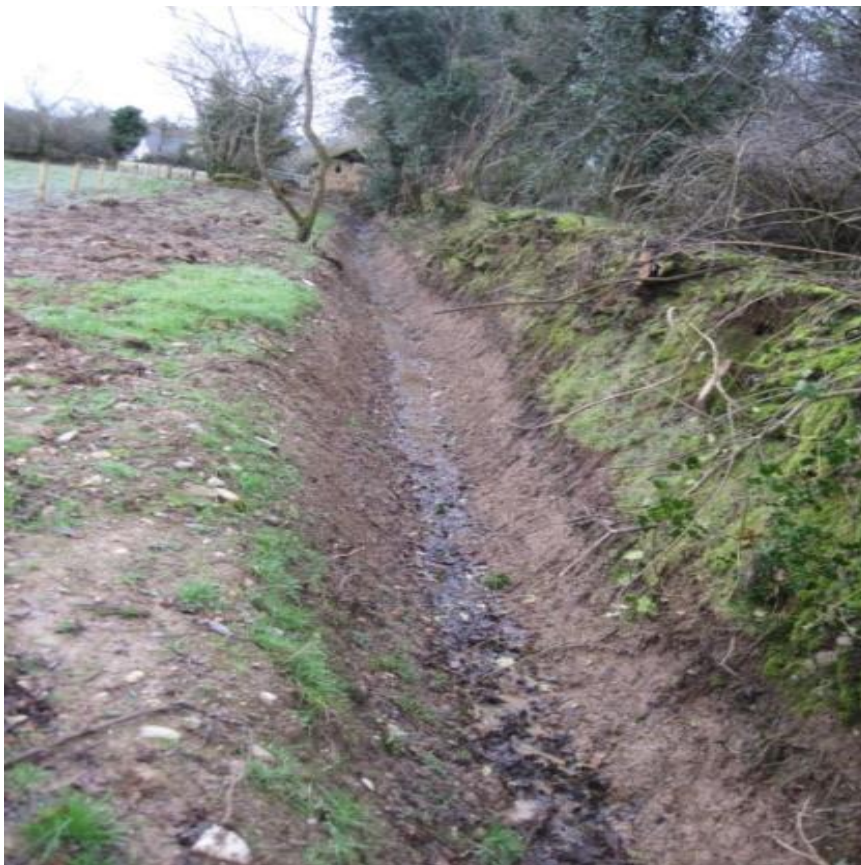
Figure 2-6: Recent dredging – temporarily exposes banks to sediment loss and removes vegetation which may have anchored sediment (Photo: Mairead Shore).
