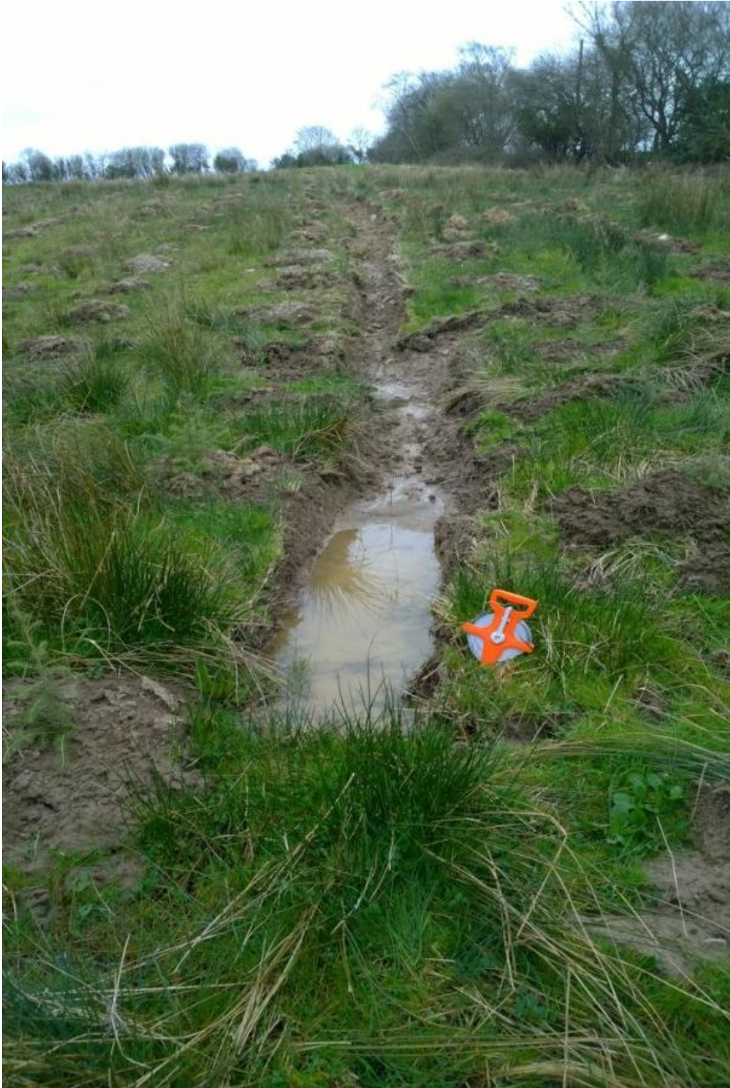
Figure 7-1: An appropriate silt trap at the end of a mound drain, on a newly developed afforestation site. The mound drain ends at the aquatic buffer zone with a vegetated, uncultivated buffer between the end of the drain and the waterbody (Photo: Forest Service, DAFM).
