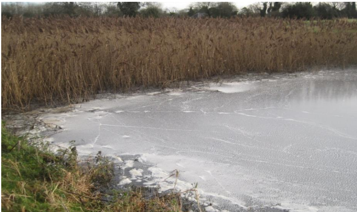
Figure 11-5: Constructed wetland receiving wash-down effluent from a food processing premises. Note detergent-type suds. The wetland was not providing adequate treatment of the effluent in this loading scenario resulting in a polluting input to surface waters, characterised principally by high ammonium in the discharge (Photo: Emmet Conboy).
