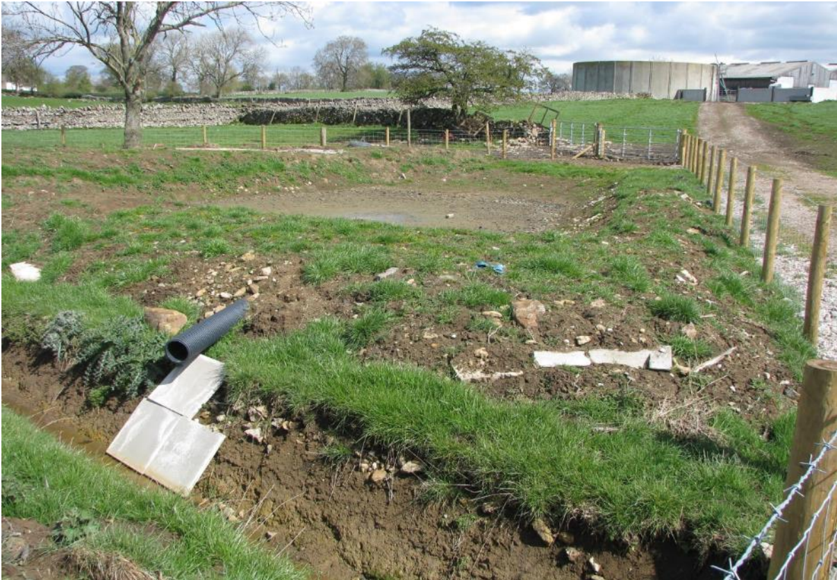
Figure 2-33: Runoff from this farm road is channelled into the sediment trap on the left (Photo: Donal Daly).
