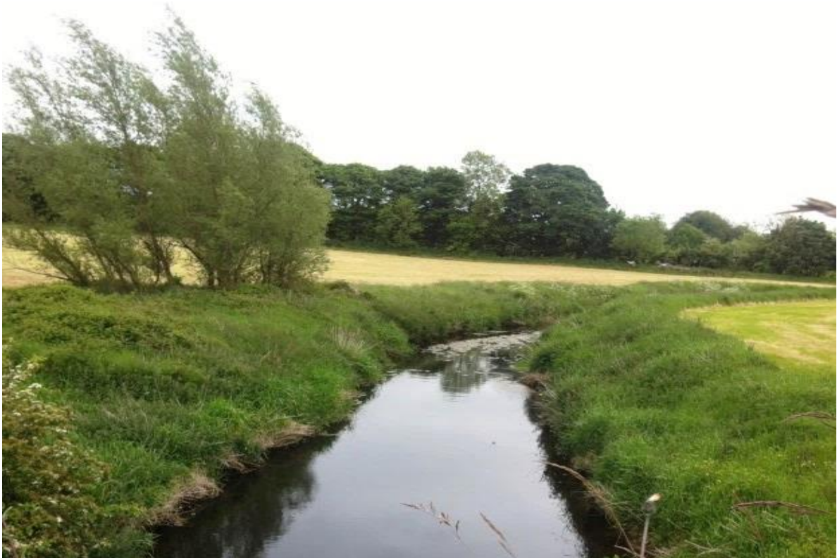
Figure 3-1: Example of a river that has undergone channelisation. Note the limited riparian vegetation along both banks and how the channel is disconnected from its floodplain (Photo: Emma Quinlan).
