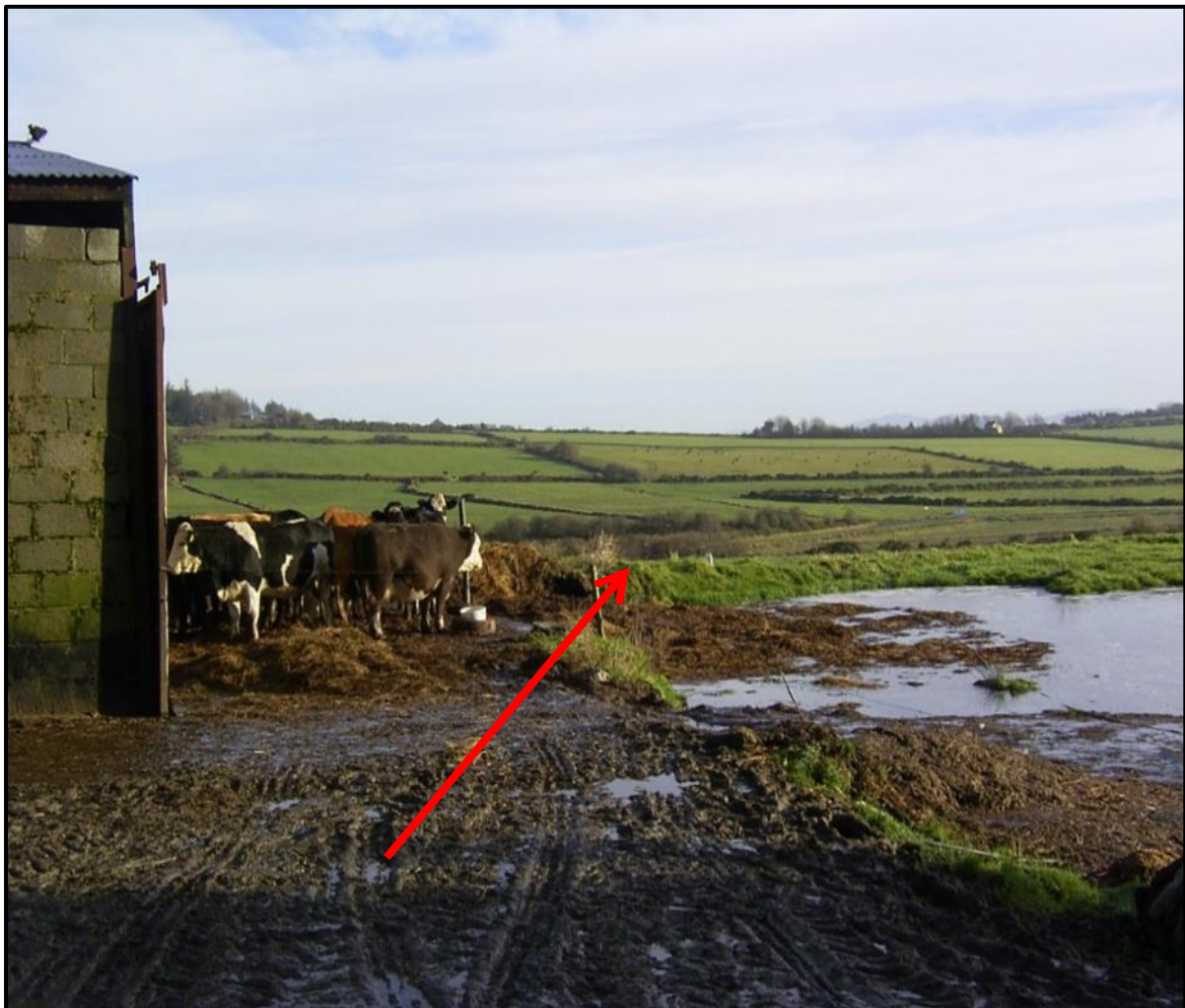
Figure 2-21: Earth lined slurry store (Photo: Andrew Holmes).
