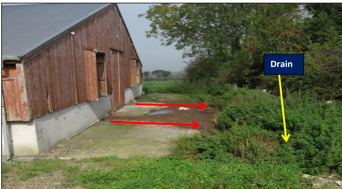
Figure 2-44: Effluent is flowing into the drain because there is no collection tank at the back of the chicken house (Photo: Andrew Holmes).
