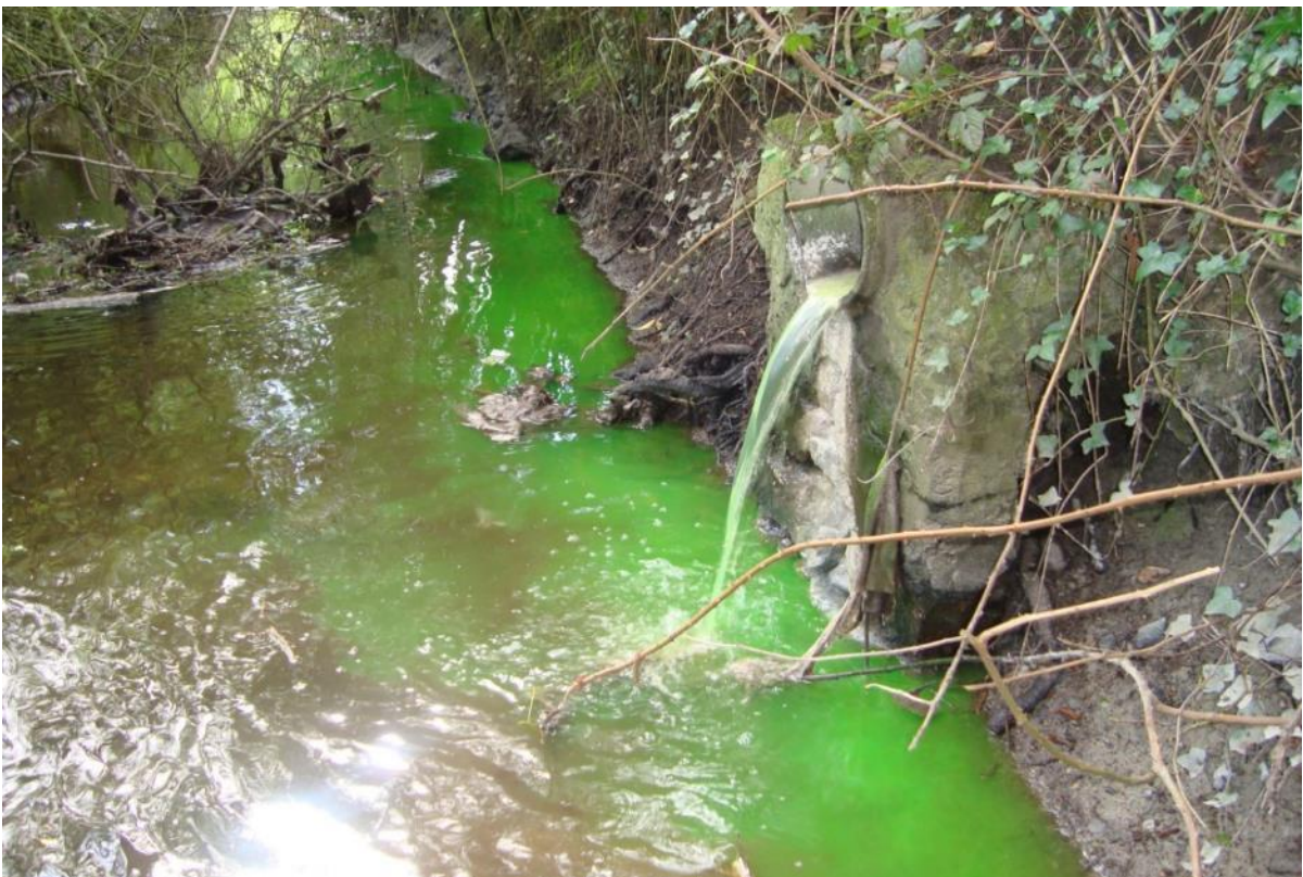
Figure 4-15: Bad Practice – Receiving water example of a direct discharge from a storm water network in low flow conditions (Photo: Joan Martin).
