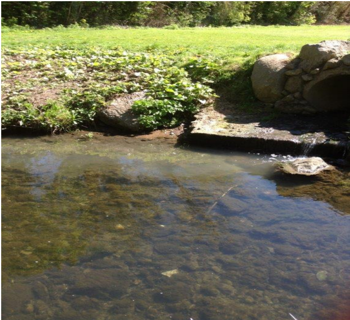
Figure 5-6: Characteristic grey cloud of misconnections entering the Shanganagh River (Photo: Paul Buggy).
