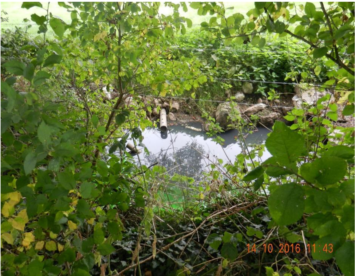
Figure 6-8: Bad Practice – Piping of “greywater” to watercourse (Photo: Joan Martin).
