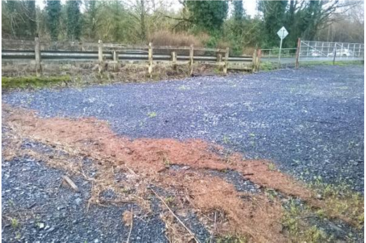
Figure 7-9: Evidence of a flooding event reaching a forest road (Photo: Forest Service, DAFM).
