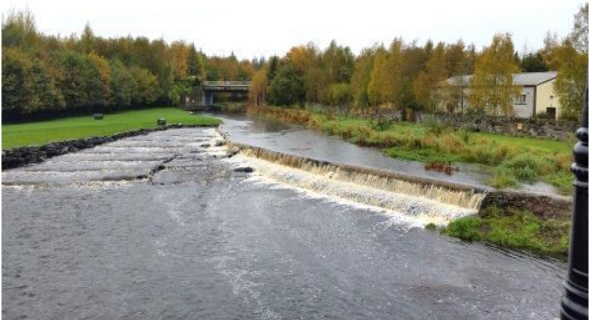
Figure 3-5: Example of a weir with a rock ramp (visible along the right bank) to allow fish passage (Photo: Emma Quinlan).
