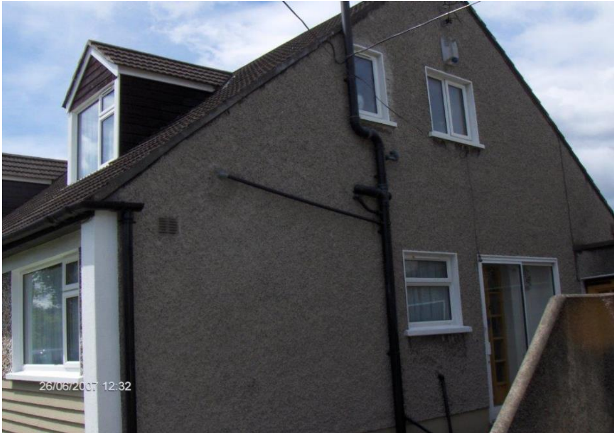
Figure 5-2: Correctly Plumbed (Photo: Tony Falkiner).
