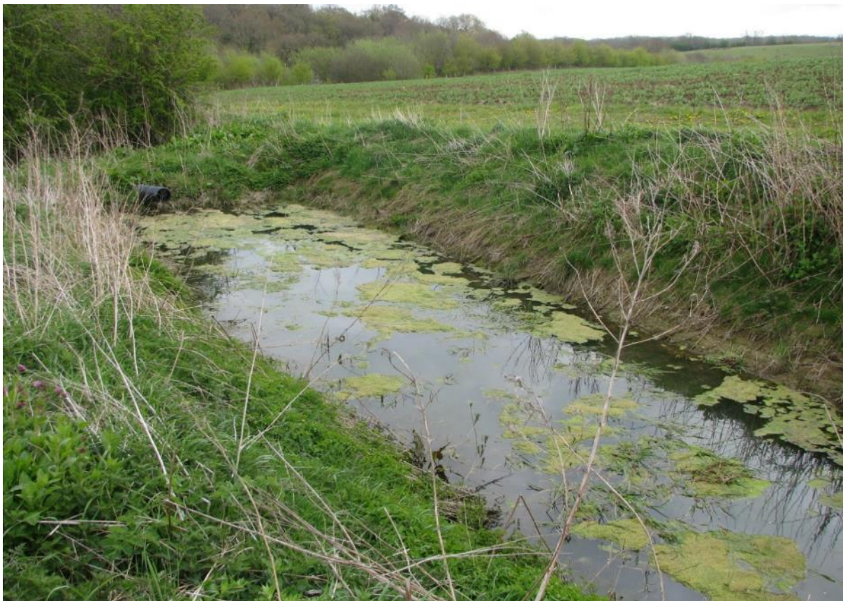
Figure 2-46: Pond constructed on a small stream to trap sediment in a tillage area (Photo: Donal Daly).
