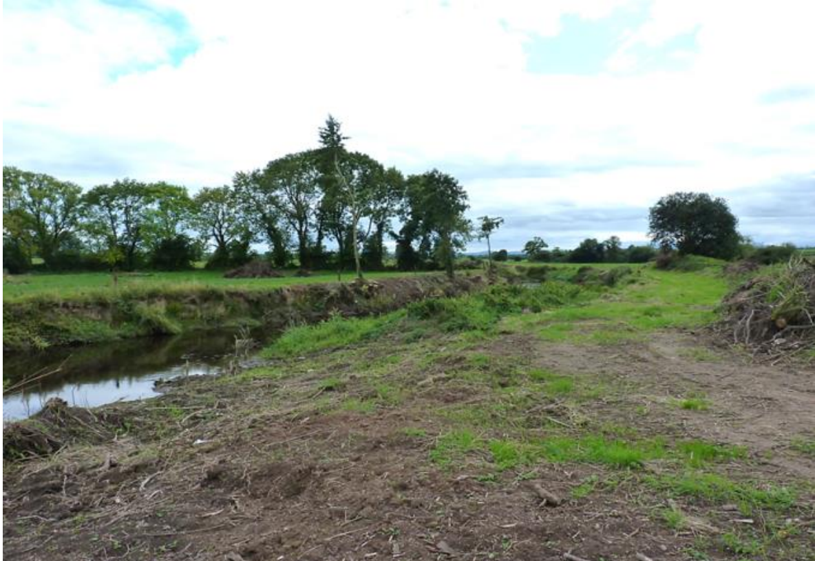
Figure 3-2: Example of a river that has undergone channelisation. Maintenance has led to the disturbance of both banks and complete removal of riparian vegetation (Photo: Emma Quinlan).
