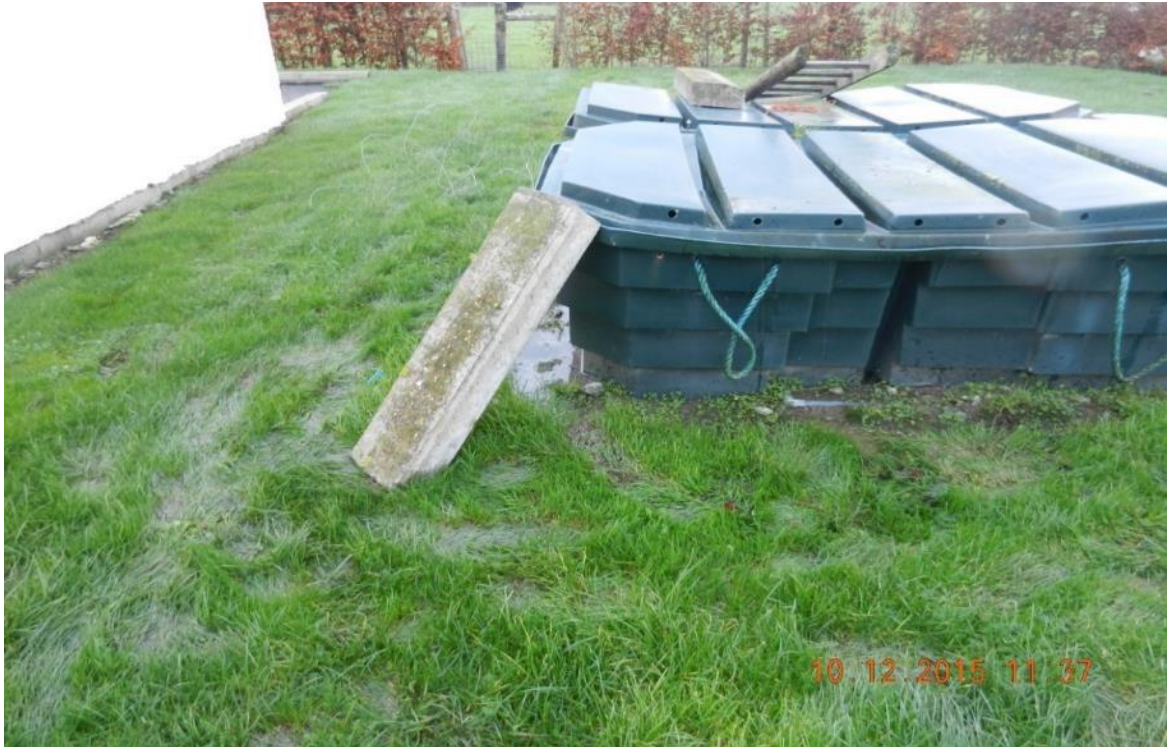
Figure 6-4: Bad Practice – Ponding of partially treated effluent from treatment system (Photo: Joan Martin).
