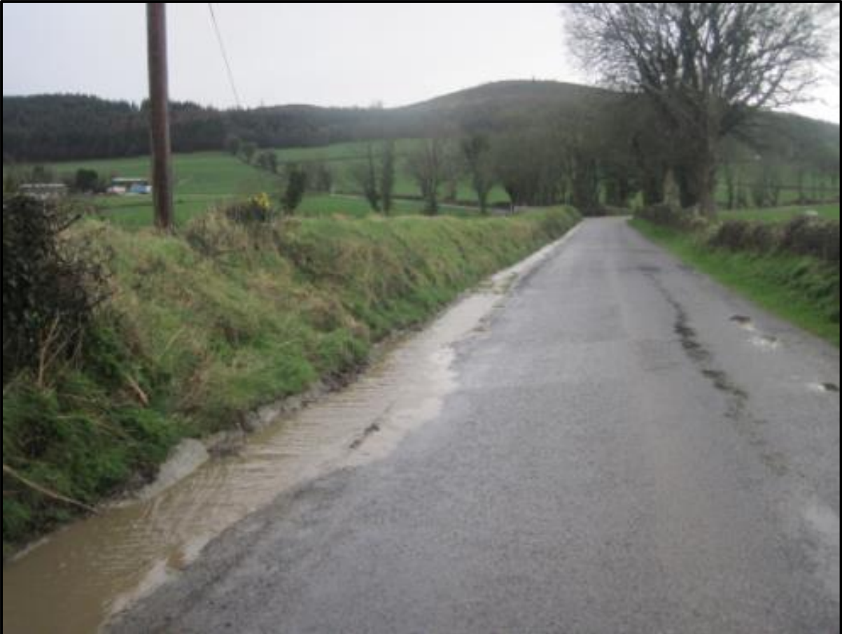
Figure 2-31: Runoff from a farm passage way onto a public road, which acts as a flowpath to an adjoining stream (Photo: Andrew Holmes).
