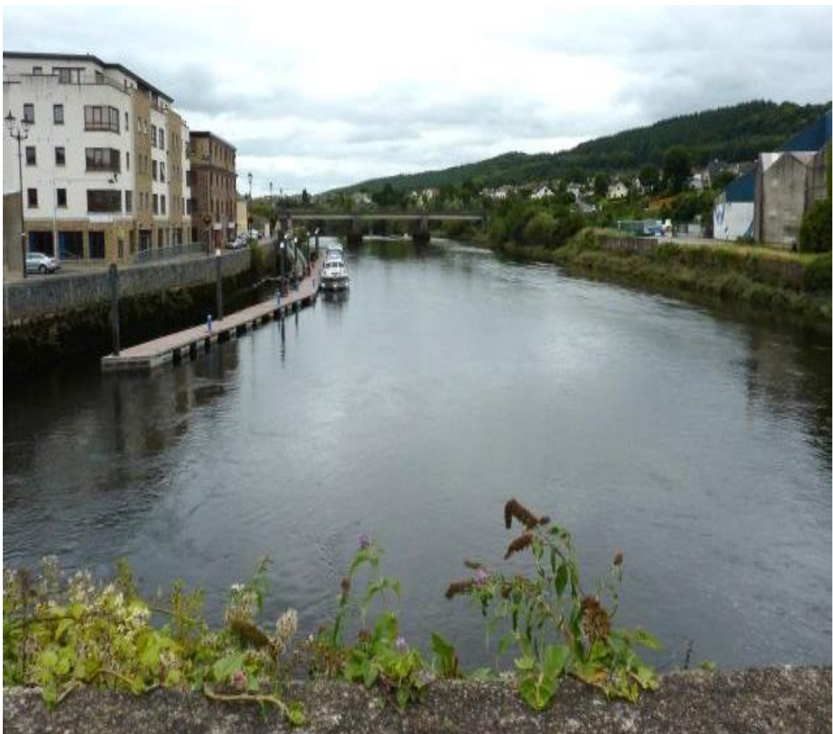
Figure 3-11: Example of the use of flood walls as flood protection (Photo: Emma Quinlan).
