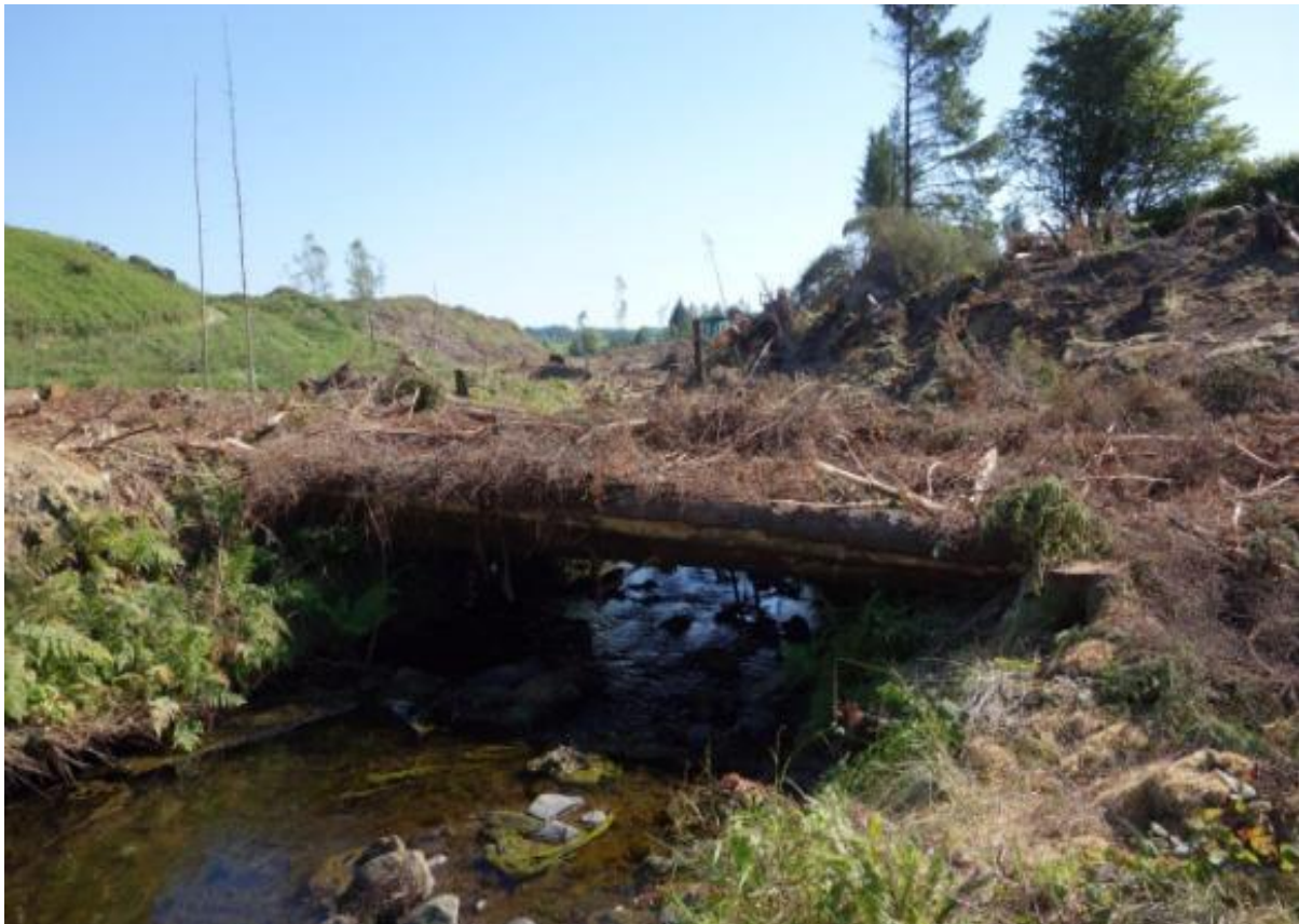
Figure 7:16: Example of a log bridge used for timber forwarding on a harvesting site (Photo: Forest Service, DAFM).
