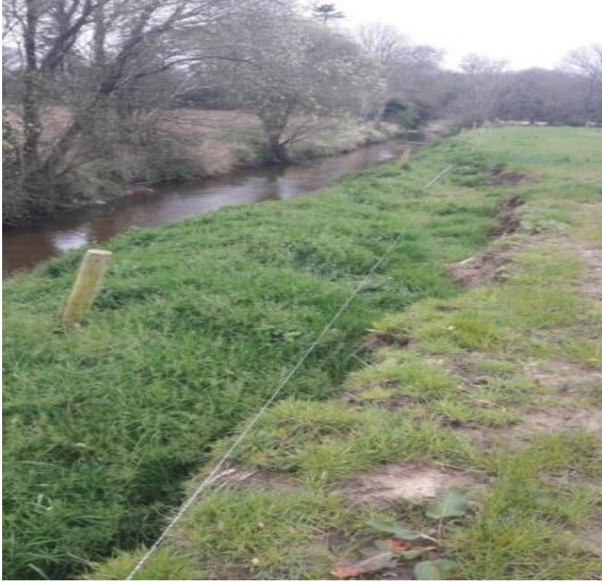
Figure 2-5: Bank collapse—delivers sediment to river (Photo: Mairead Shore).
