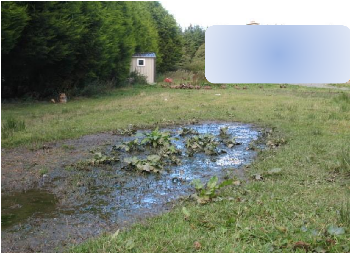
Figure 6-10: Bad practice due to inadequate percolation and ponding (Photo: Andrew Holmes).
