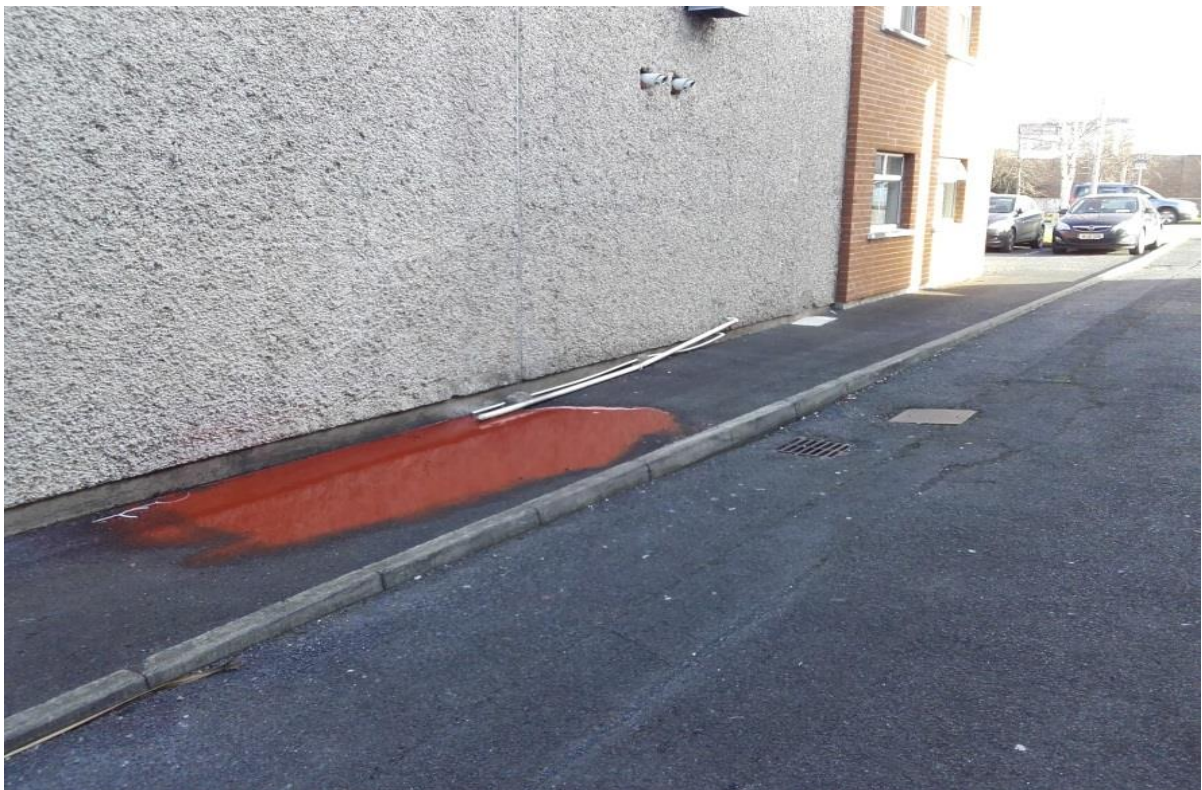
Figure 5-5: An Industrial Estate. Printing machine outlet directed onto the footpath eventually making its way to the surface water gully and to the local stream (Photo: Gerry Cullen).
