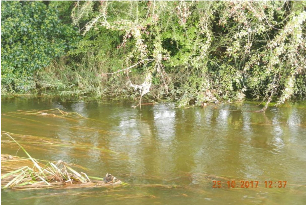
Figure 4-9: Bad Practice – Note “ragging” on the lower branches of trees on river banks and the excessive eutrophication may indicate that unscreened storm water is being discharged to the receiving water (Photo: Joan Martin).
