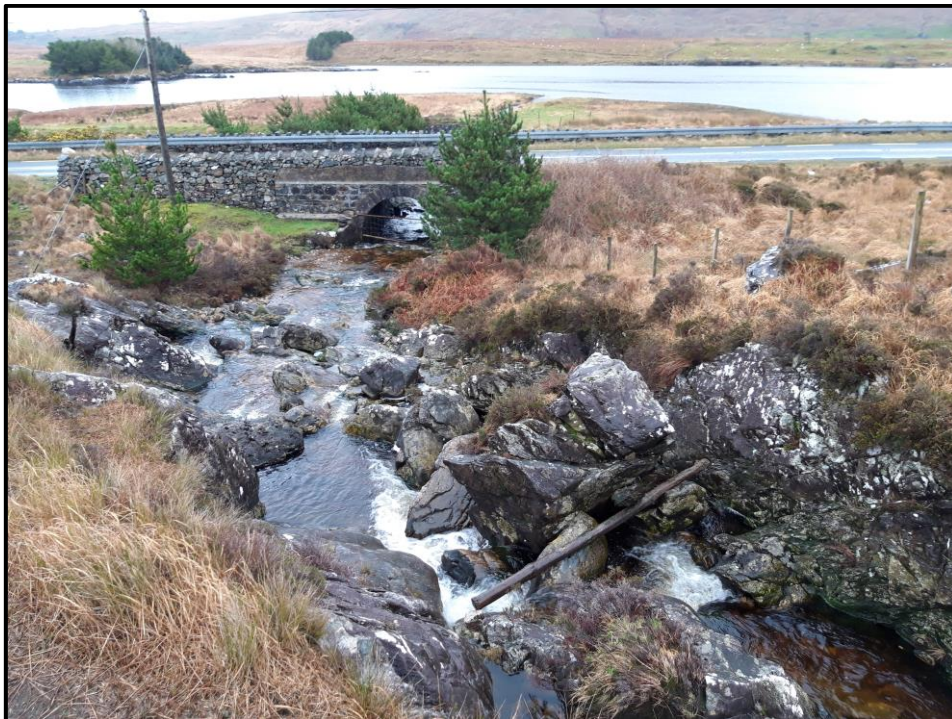
Picture upstream of the EPA monitoring station (RS31R010100) at Bunsannive Bridge on the N59
