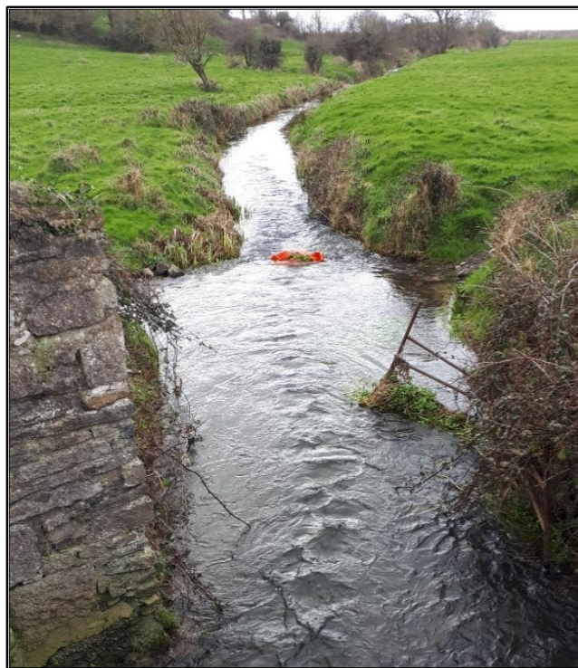
Tyshe Bridge, looking west, February 2020.
