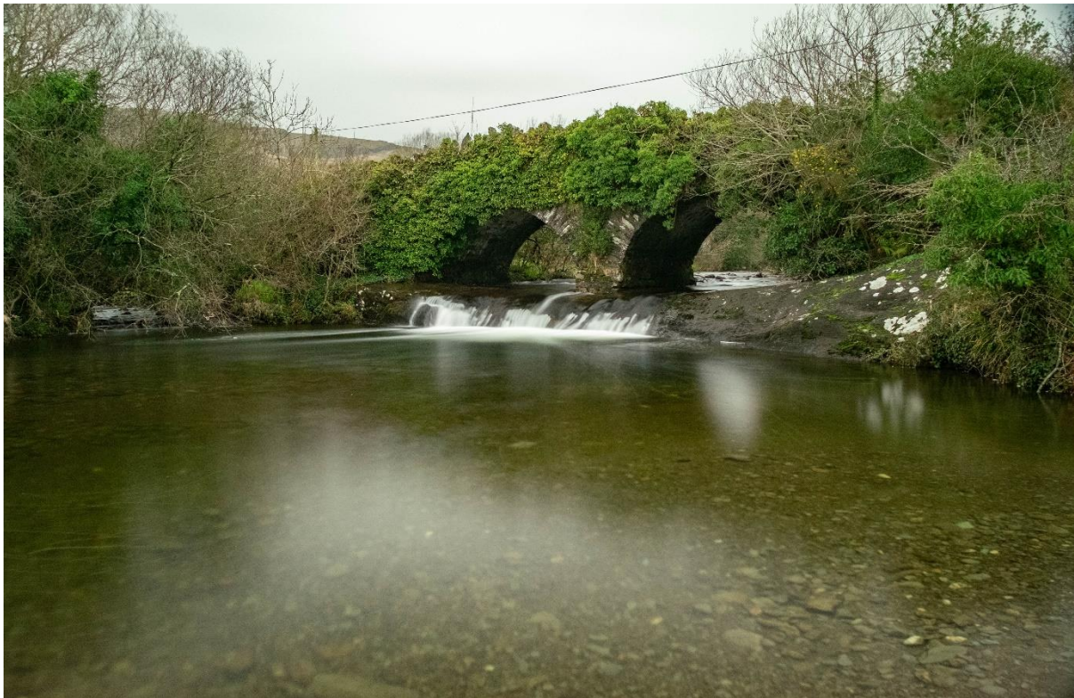
Inchintaglin Bridge Adrigole_010 taken on 13/02/2019
