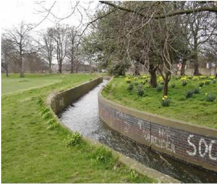
Prior to works part of the channel through Inch Park was brick lined – April 2006
