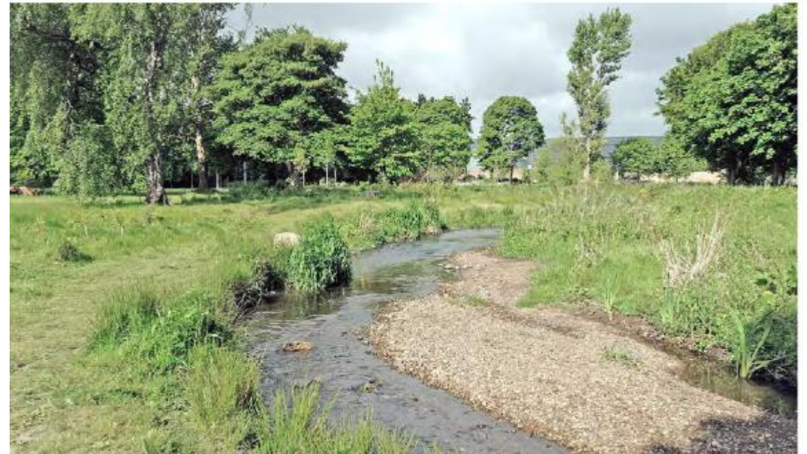
The new course of the Braid Burn through Inch Park after two years. Marginal vegetation has established well and natural processes have enhanced the
